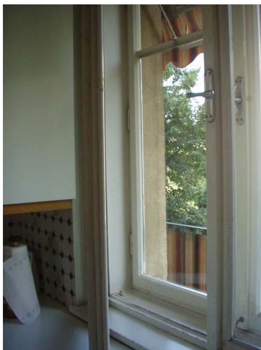
View to the garden – walls are not insulated
